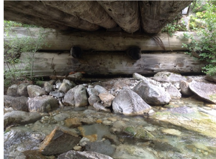
Right Bank Abutment when facing downstream
