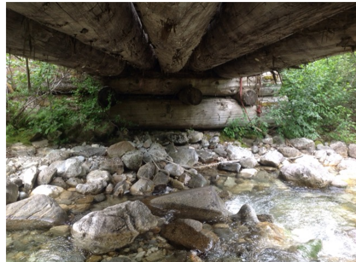
Left Bank Abutment when facing downstream
